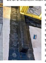
dunked the cut ends in preservative and we used our nail gun, for the first time, to put it together in sections. The gun is a bit unwieldy, but is quite fun to use and we got 500+ nails done in an hour and a half. The next day we stood the sections up, nailed them together and screwed them down to the foundation blocks. And that was that.
