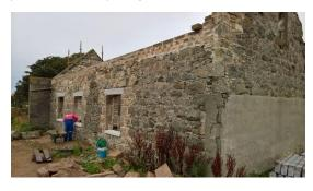
**Wallheads** – we finished the four courses of concrete blocks along the east wing walls, that raise the roof to the designed height. Over that we
