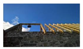
Raised tie trusses on the north wing – our last day on site was getting Ric set up to work on his own. We got the first truss prepared, lifted over the wall and manoeuvred into position at the join with the east wing, nailing it to the ends of the
