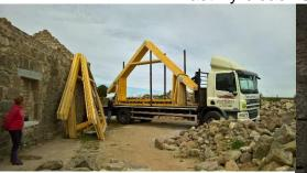
simple as it sounds and it took us longer than we expected, but we got there. We used angle-brackets to fix the first one to the gable wall, then battens across the truss
