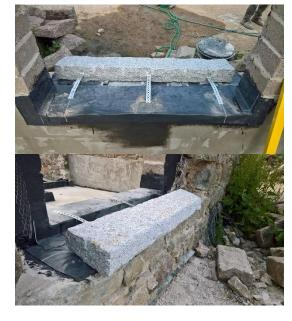
with a gap that we filled with concrete. We waited another day for it to go off, then built up courses of granite rubble above the lintels, up to the original wallhead. We worked on the other two window openings at the same time. By the time I drove back southall three had sills, quoins and lintels.
