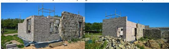
Concrete blocks: The rest of the time we spent building up concrete blockwork, mostly on the first gable-end we demolished, in the west wing. We just about got it all up to upstairs-
