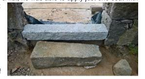
**Door sills:** Ric experimented with the kitchen door onto the courtyard. After much measuring up, he chiselled out grooves in the quoins at the base of either side of the door opening, cut one of Jill & Andy Walker
