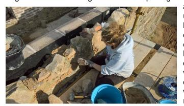
are now windows. up to sill height. Ric has rebuilt a derelict doorway, reinstated existing granite lintels above the door and adjacent window and we completed the walling above, to roof-height. Another
