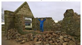
took out the pillar of stonework in between. This turned out to be good and bad. Good, because chunks of the wall were in shocking condition, with cement, brick rubble and even a 1m wooden plank embedded in it. Bad because, by the time I had pulled out all the rubbish and wet, decomposed, lime mortar, the opening was enormous and almost went up to the next opening in that wall. A case of being cruel to be kind!
