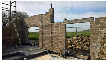
over the original building, to give us headroom on both floors of east and west wings. We have laid all the concrete blockwork for this that we can and can accurately measure up for roof trusses, when we are ready!
