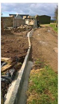
Ric was on site at the start of April and did three weeks of preparation. He got rid of our standing water with two lengths of french drain, laid a linear drain in front of our garage & front doors, cut concrete structural lintels to size and laid more concrete blockwork where we need to rebuild walling. He assembled our
