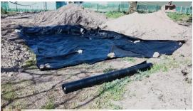
layer of weed membrane then made good with subsoil and topsoil. He laid drains up each side of the courtyard for gutter downpipes. The last job will be
