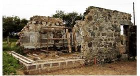
wallheads, to protect the them from the weather and to prepare for the blockwork that will support the roof trusses. I got much of the blockwork
