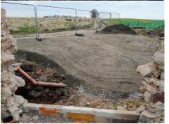
Minor flooding: We were surprised at the amount of standing water on our track as it approaches the steading and on the drive-off onto our hardstanding. Delivery trucks would get bogged down. On investigation, we found land drains that looked to have been cut through and blocked when our water supply was run to the steading over a year before. They must have backed up a head of water to the point where a spring had
