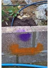
Getting final floor level marked out: We need to know exactly where our final floor level needs to be so we dig down to the right depth to lay hardcore, sand blinding and the concrete floor slab. Then we can get joists, roof trusses, doors and windows at the right levels as well. We got the level and staff out, worked out floor
