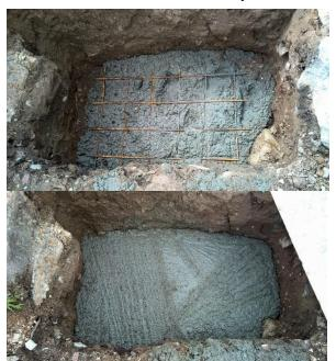
finished that then cut up the reinforcing mesh for each trench. We got some plain reinforcing bar to make pegs to hammer into the base of each trench, to mark the correct levels and depths of concrete.
