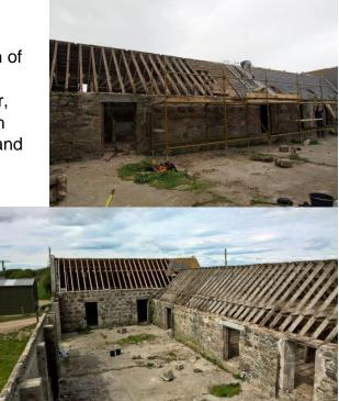
one end of a rather massive concrete lintel that is embedded at the other end into one of our gable-ends. I worried about it working loose and bringing the gable-end down with it. I worked out it was about half a tonne, so we put scaffolding under it, hired a concrete saw and cut it
